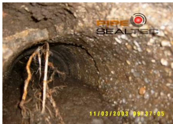
Figure 6-15 Pipe fouling
