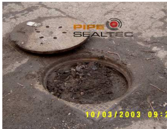
Figure 6-14 Shaft fouling
