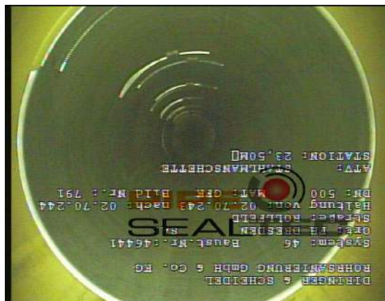
Figure 6-56 documented rehabilitation area Pipe-Seal sleeves Serial mounting
