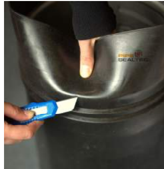
Figure 6-30 Simple cut of overlapping rubber
