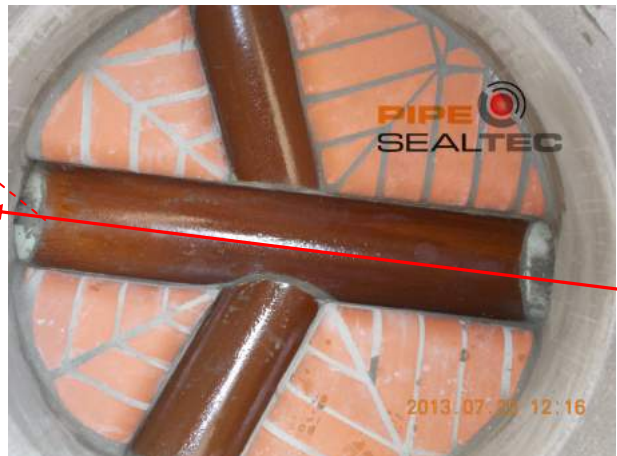
Figure 6-12 Forming of access possibilities such as channel profile and pipe connection
