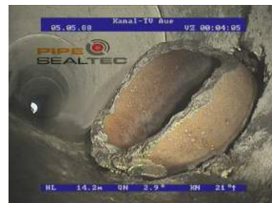
Figure 5-15 Protruding connection piece
