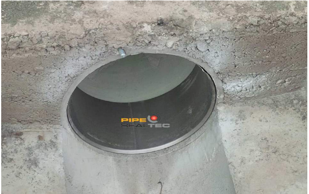
Figure 5-20 Liner connections with Pipe-Seal-End
