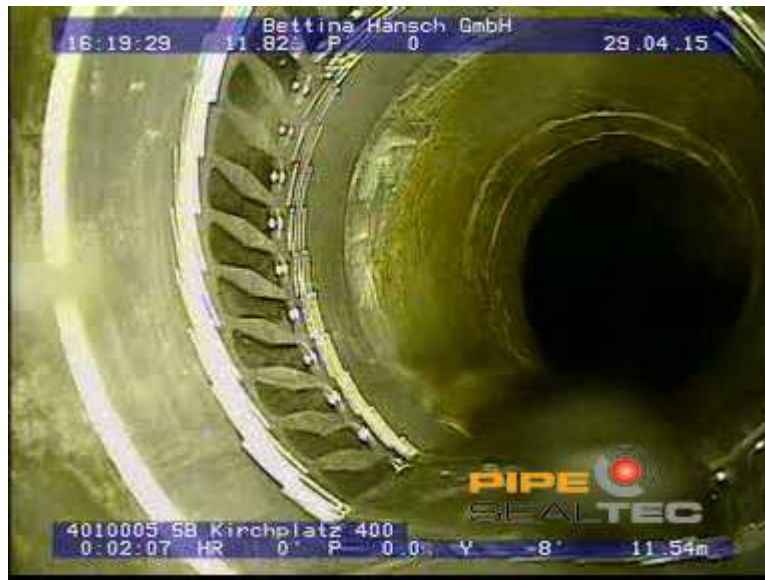
Figure 6-61 Rehabilitation with Pipe-Seal-Flex on angular offset
