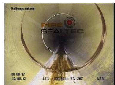
Fig. 5-13 Leaky pipe connection
