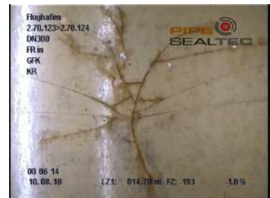
Figure 5-12 Crack formation
