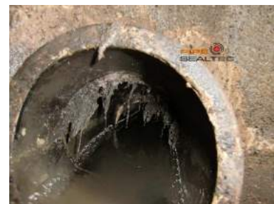
Figure 5-19 Penetrating roots
