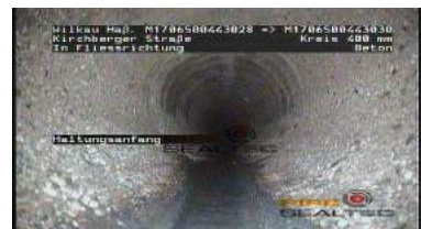
Figure 5-17 Concrete corrosion
